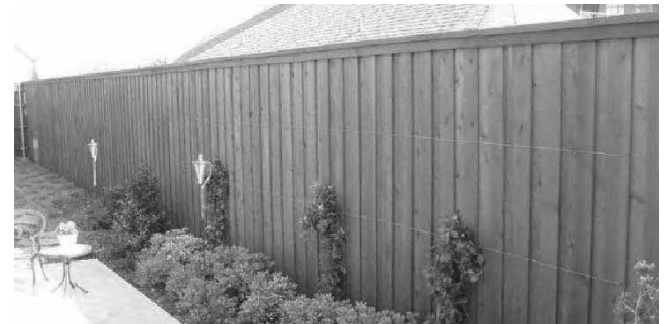
PRESTAINED CEDAR BOARD-ON-BOARD FENCE WITH TOP SIDE STRIP, TOP CAP, AND PRESSURE-TREATED KICKBOARD
