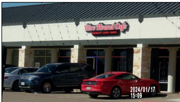
FRONT OF BUILDING (HILLTOP DR)
