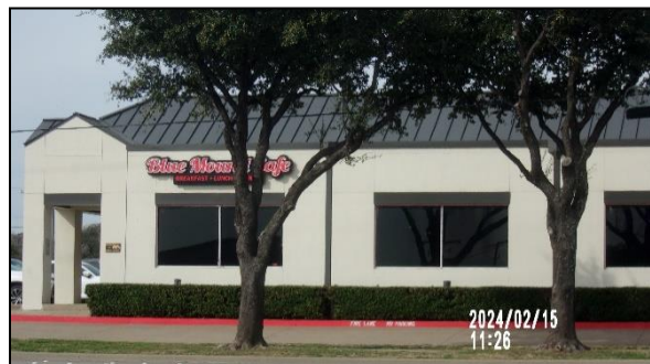
SIDE OF BUILDING (RUFESNOW DR)
