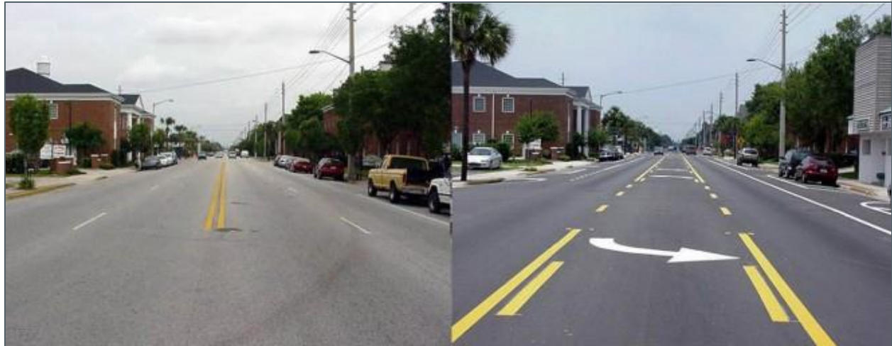
Road Before and After Restriping
