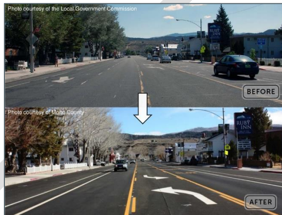
Before and After Restriping
