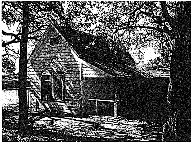
The Hightower/Autrey House, dating from the 1880s, is the last 19 th century historic residence in the city, and represents an excellent and rare example of this style and type of farmhouse.
