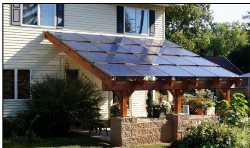
ATTACHED SOLAR PERGOLA
