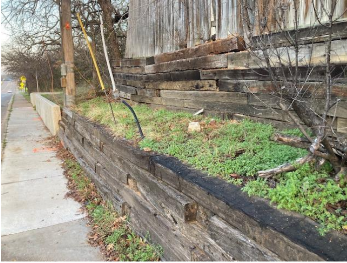
View looking west of retaining wall along south property margin
