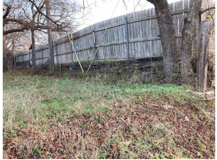
View of retaining wall along west property margin
