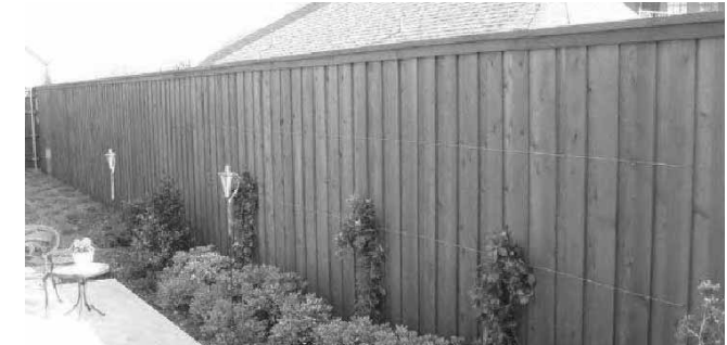
PRESTAINED CEDAR BOARD-ON-BOARD FENCE WITH TOP SIDE STRIP, TOP CAP, AND PRESSURE-TREATED KICKBOARD
