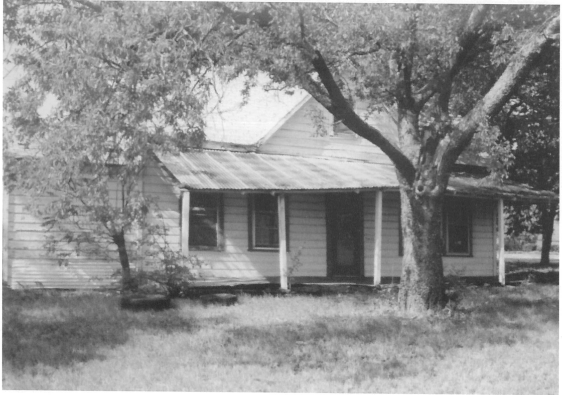
Hightower/Autrey house at 6725 Smithfield Road. Jimmy Hightower probably built this house for his son, L. A. Hightower, around 1880. This was the home of L. A. Hightower until 1918 when the Bud Autrey family purchased it. This house is one of the oldest in the Smithfield area. Photo taken 1998.
