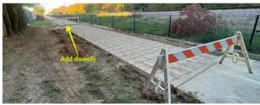
Concrete repairs have been made to one section of the Cottonbelt Trail north of Eden road and will be followed by a drain in this section to eliminate standing water faster after rainfall. Walkers Creek Park will also be receiving concrete repairs in the coming month as soon as additional bids are received.
