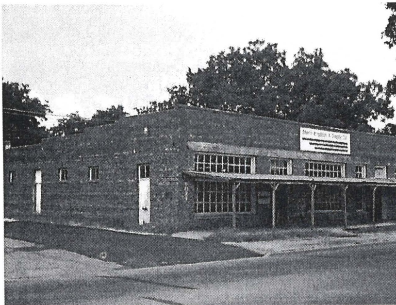
Smithfield Feed Store - This structure is located at 8021 Main Street and was built in 1926. It is believed to be the oldest remaining commercial building.
