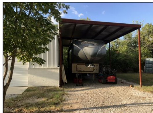
VIEW OF BUILDING IN 2022 (PRIOR TO REMOVAL OF CARPORT)
