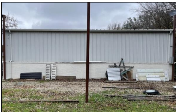
SIDE VIEW OF EXISTING BUILDING
