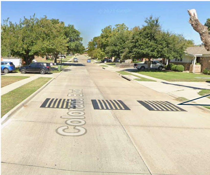
Speed Cushions installed March 2018
